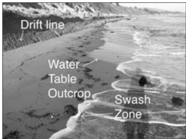
Figure 2. This view looking east along an old concrete seawall on the Gaviota coast at low tide illustrates the attenuation of intertidal zones on a beach seaward of coastal armoring.
